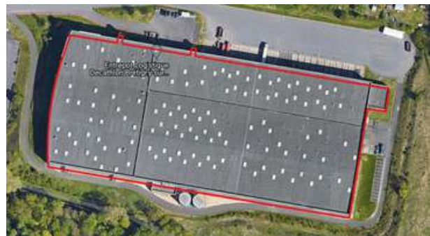
Figure 3.5: Decathlon Warehouse south of Paris.
